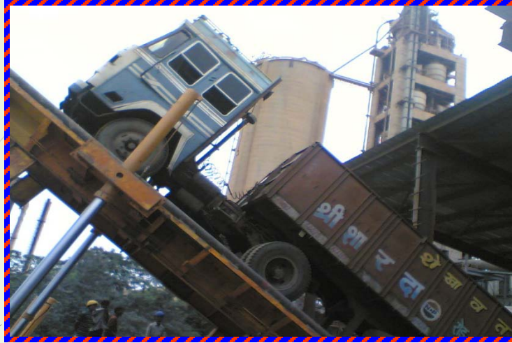
Step – 1 Unloading of RDF (Refuse Derived Fuel) into hoppers)
