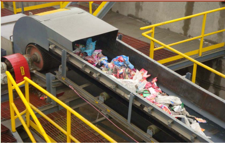
Feeding Of Plastic Waste Into The Shredder
