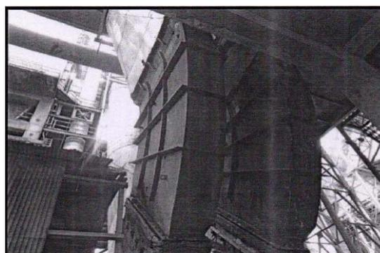
**Figure 19 Raw Mill Fan Inlet Duct**
