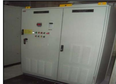
**Figure 16 VFD Line-2 Pre-heater ID Fan**
