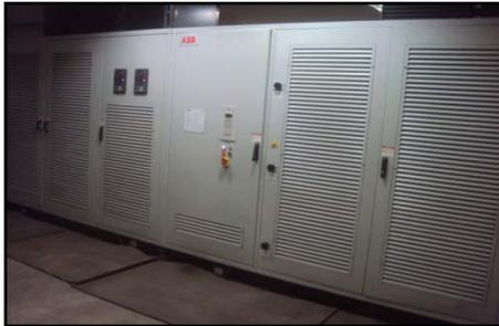
**Figure 15 VFD for Line-2 Cement Mill bag filter fan**
