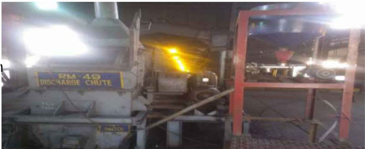
Figure 30: Arrangement showing feeding of Thermact (catalyst) inside the kiln
