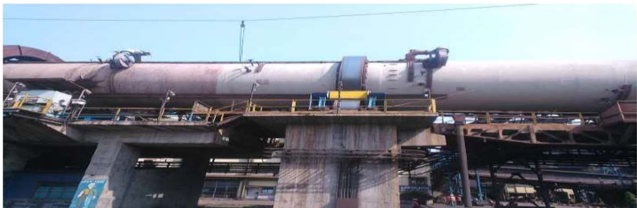
Figure 29: Application of Heat Shield Paint on the outer surface
