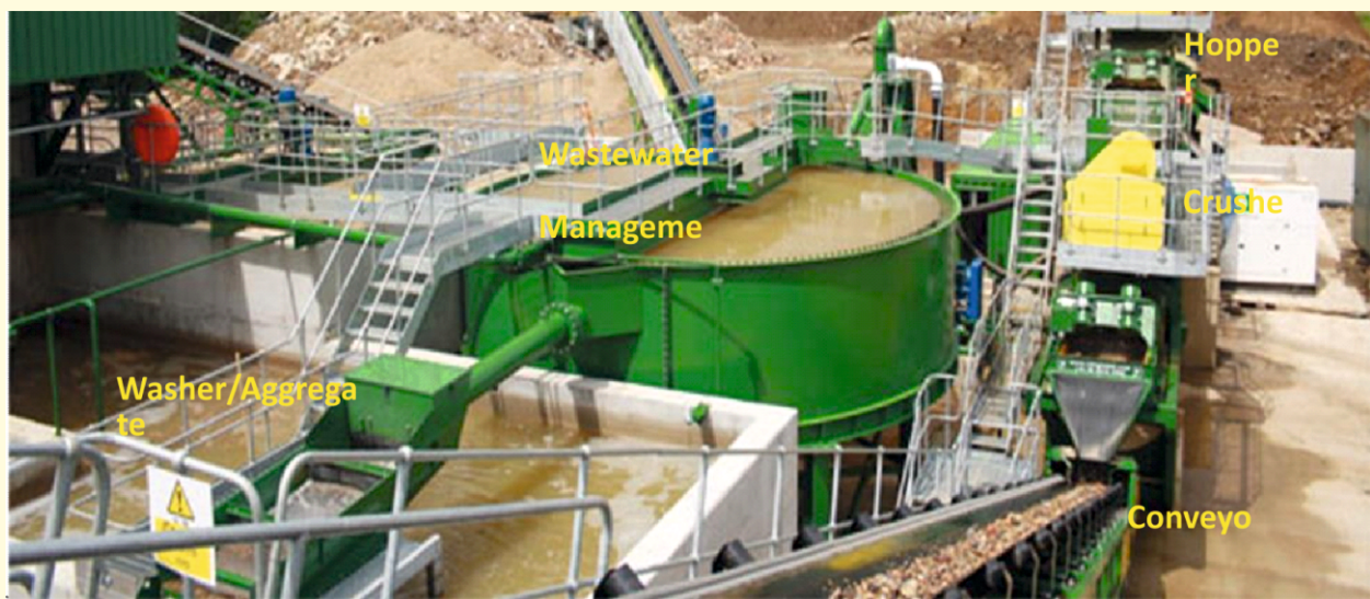
Figure 6.4.1 - C&D Waste recycling plant in Delhi
